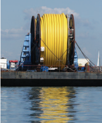
Pipe laying in the Solent
