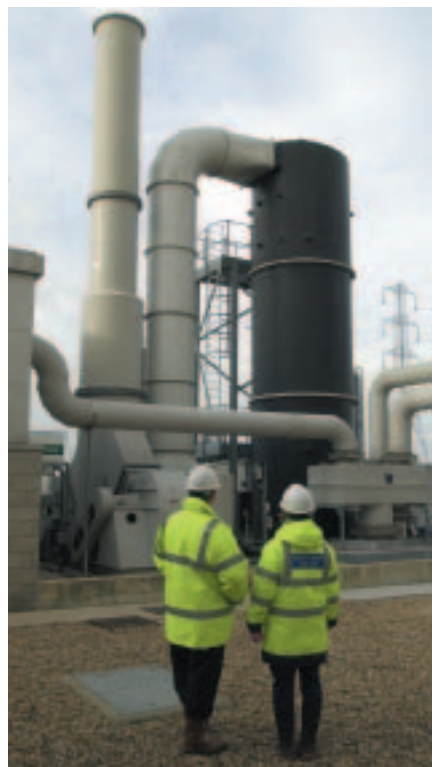
Odour control systems would be installed at both Ashford and Aylesford to remove smells
