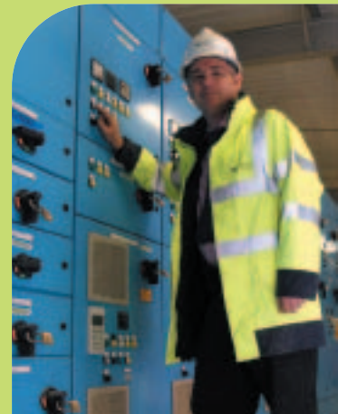
Project Manager Barry Knight inside the new microfiltration plant at Otterbourne Water Supply Works
