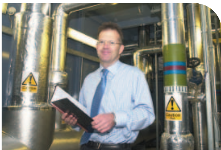
Inspecting part of the Combined Heat and Power plant at Goddards Green in Sussex
