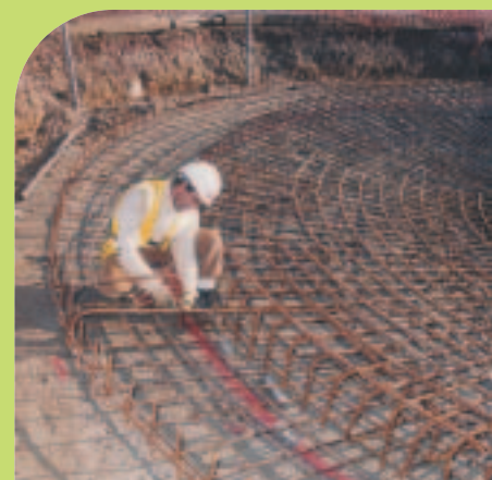
We will renew, renovate and refurbish treatment works during 2005-2010
